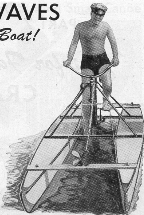
Pontoons for your bicycle boat can be made as shown or adapted from war-surplus airplane belly tanks
